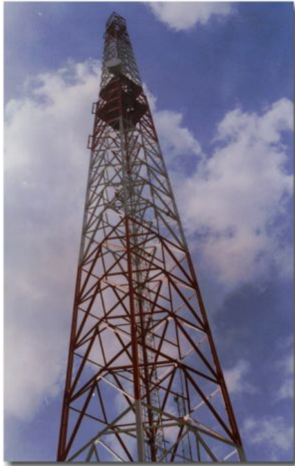
80m Backbone Tower - Nigeria
